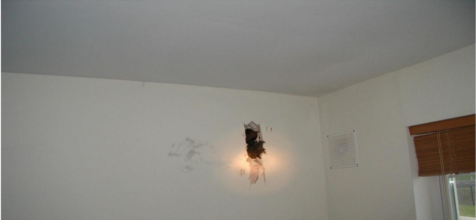
***Fire within the cavity of the gable end wall was not evident until part of the plaster slab was removed by fire fighters. Note no evidence of fire or smoke staining within the room itself.***
