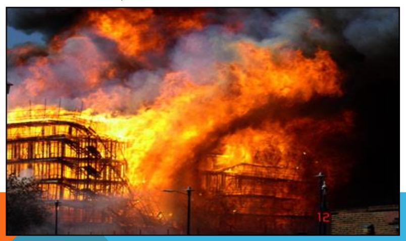
**Unprotected Attic Space – No Fire Stopping / Walls between Blocks:**
