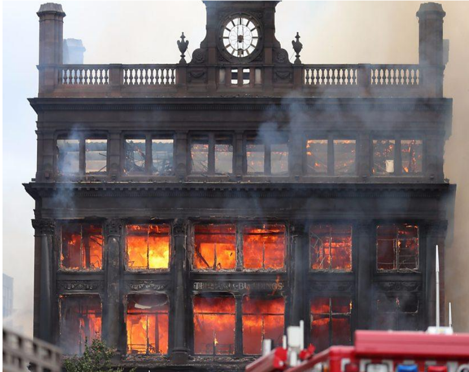
Primark fire: August 2018, Belfast
